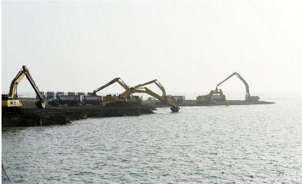
Figure 13: Figure 1.1: Construction work on New Baku Sea Port
